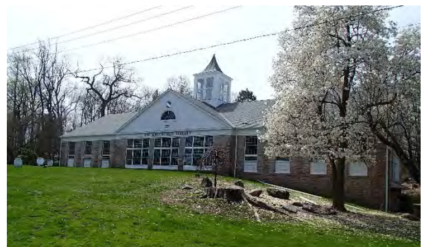
Brookfield Library, 182 Whisconier Road – Image Source: Brookfield Vision
