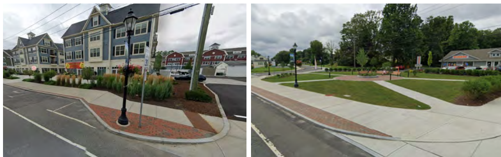
Early Phase Sidewalk Additions in Four Corners
