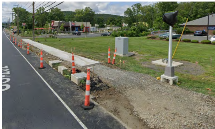
Route 202 Sidewalk Construction
